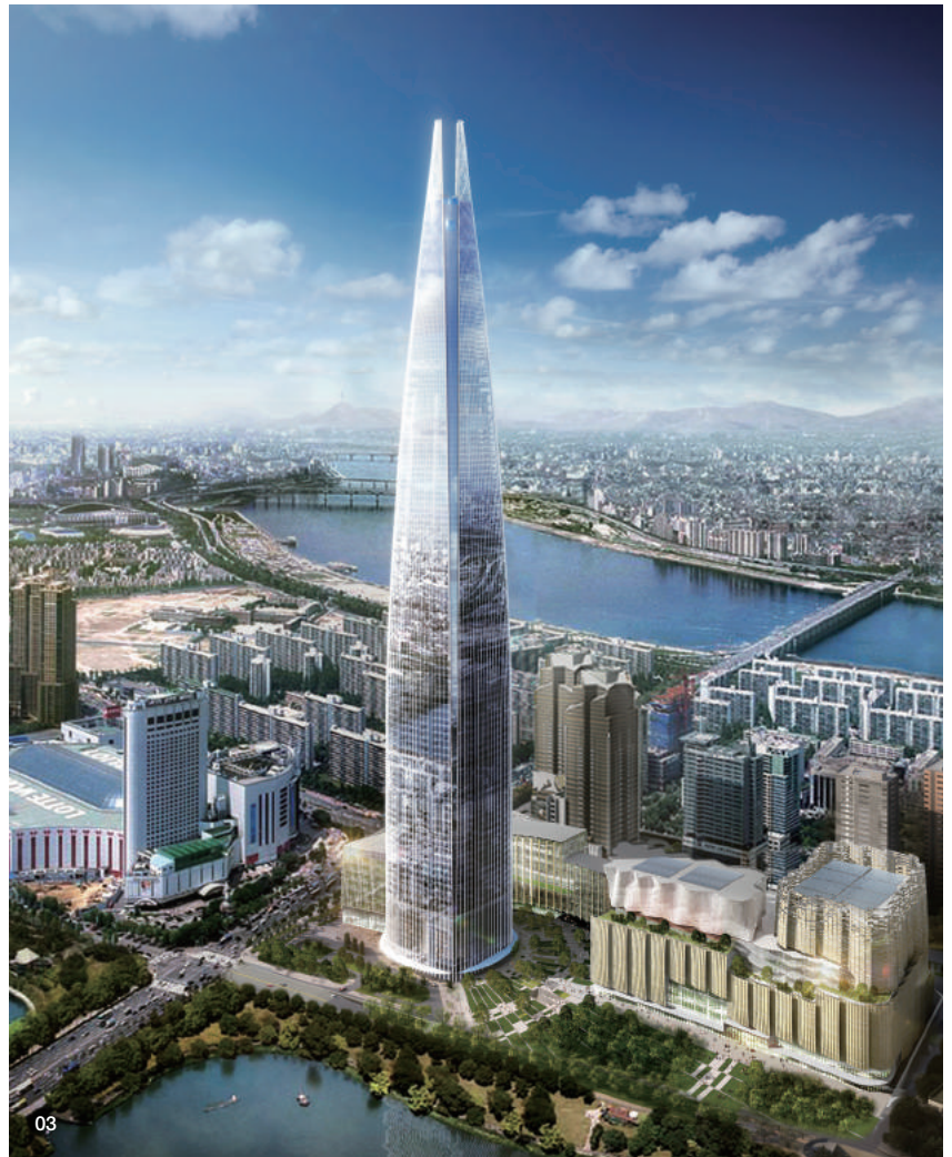
03 Lotte Tower Service : Environmental Impact Assessment Location : South Korea Client : Lotte Corporation, Lotte Shopping, Hotel Lotte
